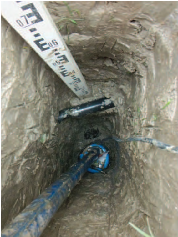
TH1 Water Main and Trace Cable
