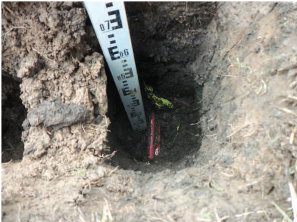
TH6E Electricity Cables
