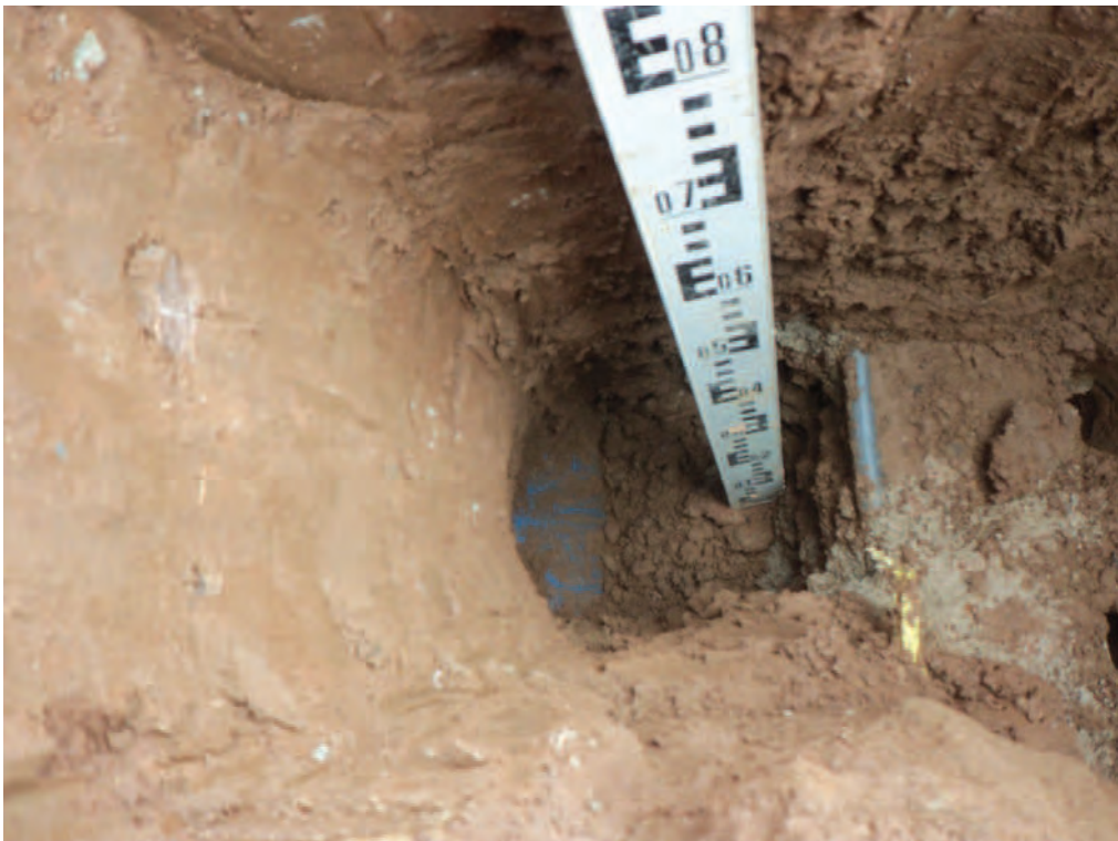
TH7 Water Main and Trace Cable
