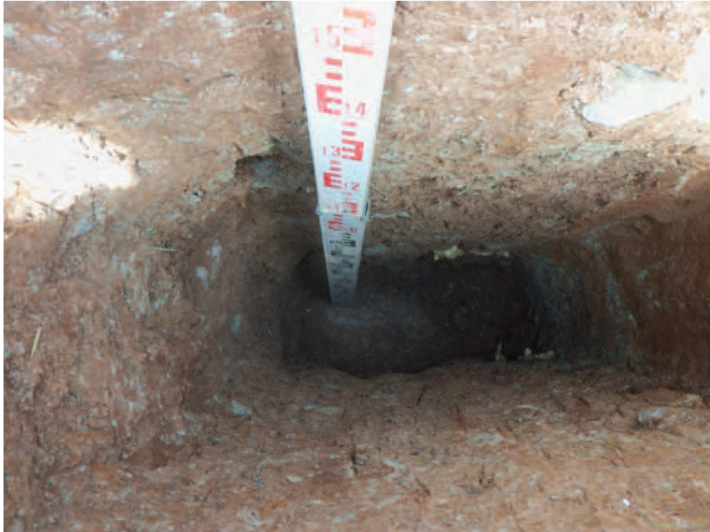
TH3 Water Main and Trace Cable
